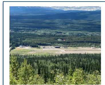
Commenced Dease Lake airstrip upgrade following award of StrongerBC grant
