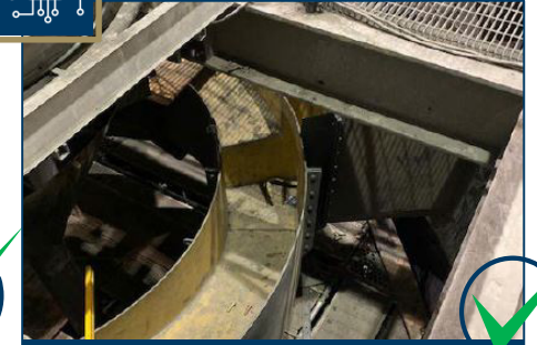
Two donut launders installed
