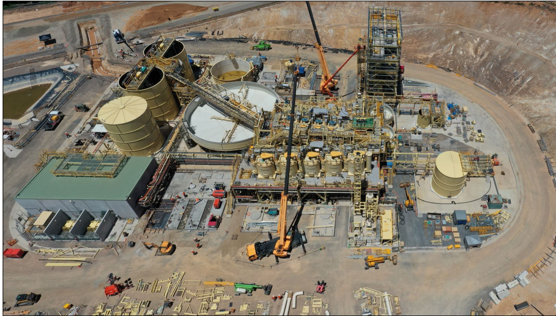
Current Progress Photo (January 2021)
