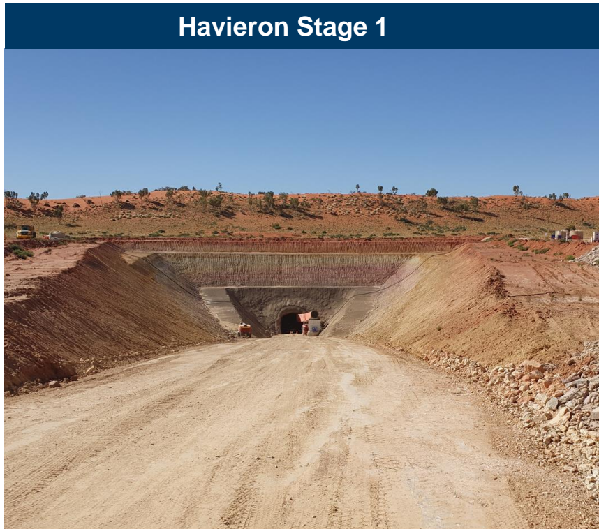
Figure 1: Havieron Exploration decline has advanced 226 metres as at 10 November 2021
