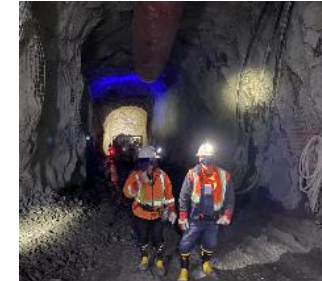
Exploration decline now progressed 765 metres as at 25 January 2022
