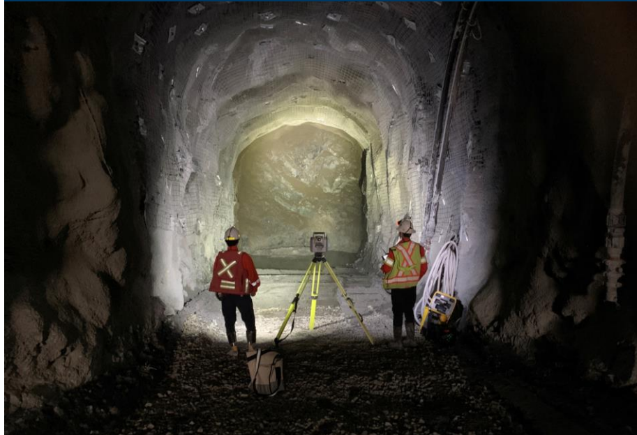
Red Chris Exploration decline has advanced 527 metres as at 10 November 2021
