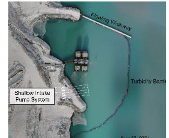
TIA Turbidity curtain installed - winter water management campaign
