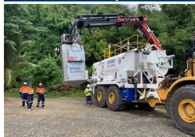
Robotic explosive placement
