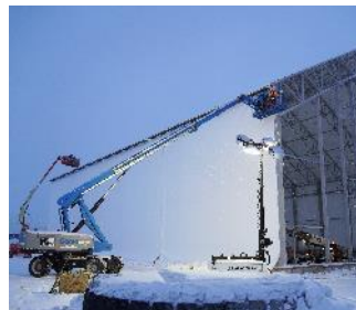
Life of Mine maintenance and warehouse facilities nearing completion
