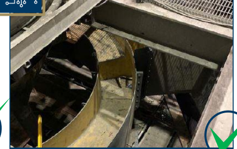
Two donut launders installed
