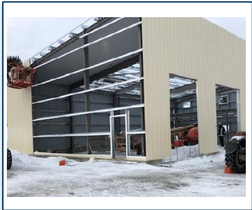
ERT Building under construction to house emergency vehicles, ERT and Iridia medical facilities
